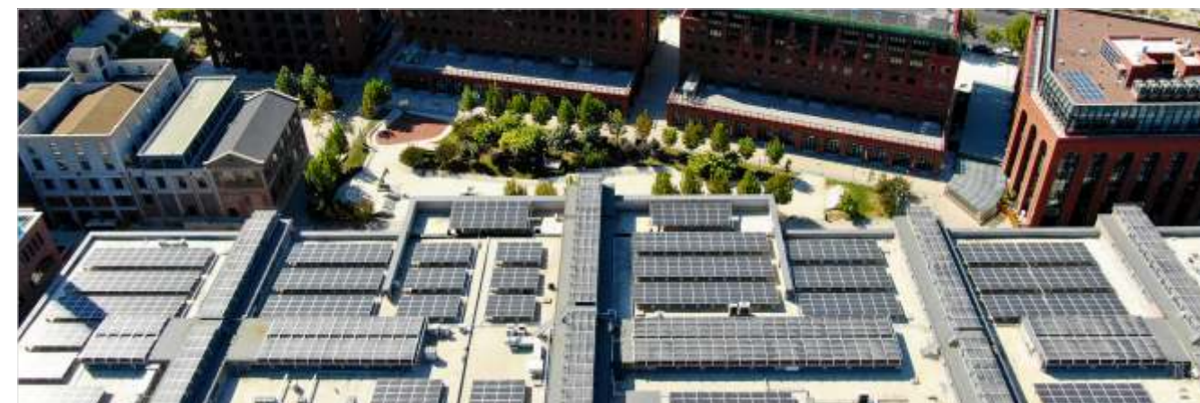
Phase I R&D and Construction Project of Tianjin Comprehensive Smart Energy Information Management and Centralized Control Platform
