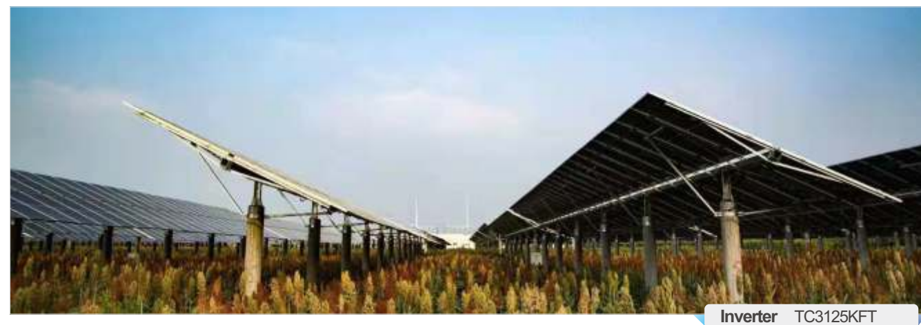
Hubei Qianjiang 100MW Photovoltaic Power Plant
