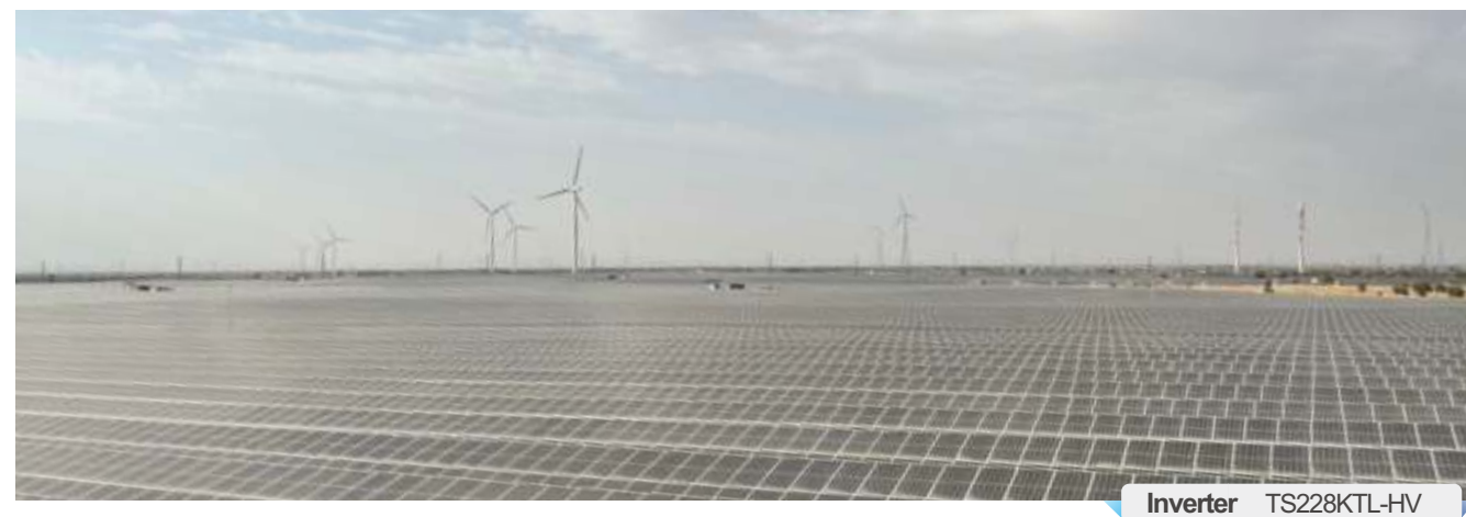
India RENEW 150MW Photovoltaic Power Plant
