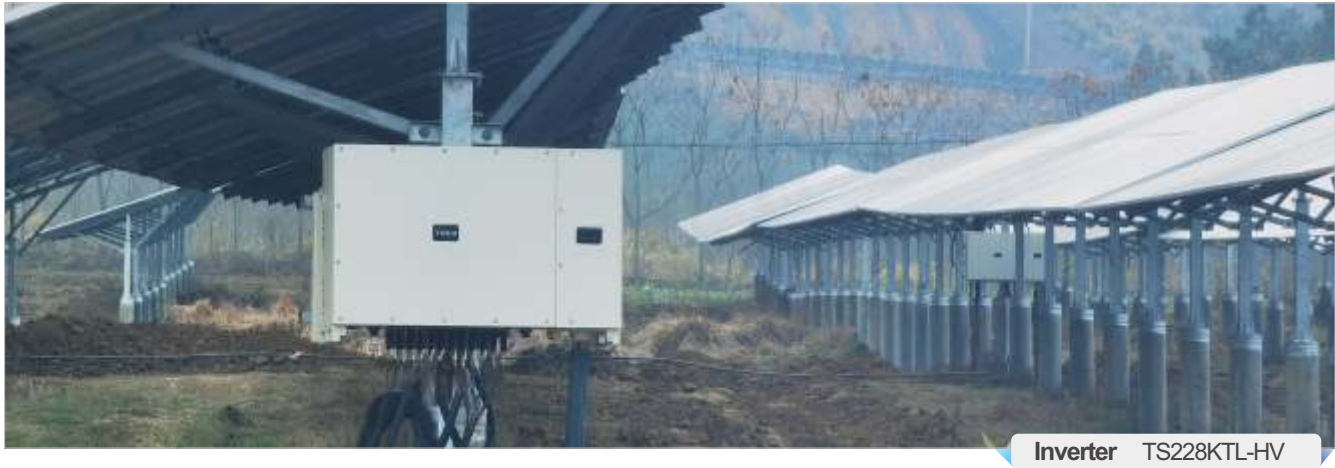
Hubei Qichun 99MW Photovoltaic Power Plant
