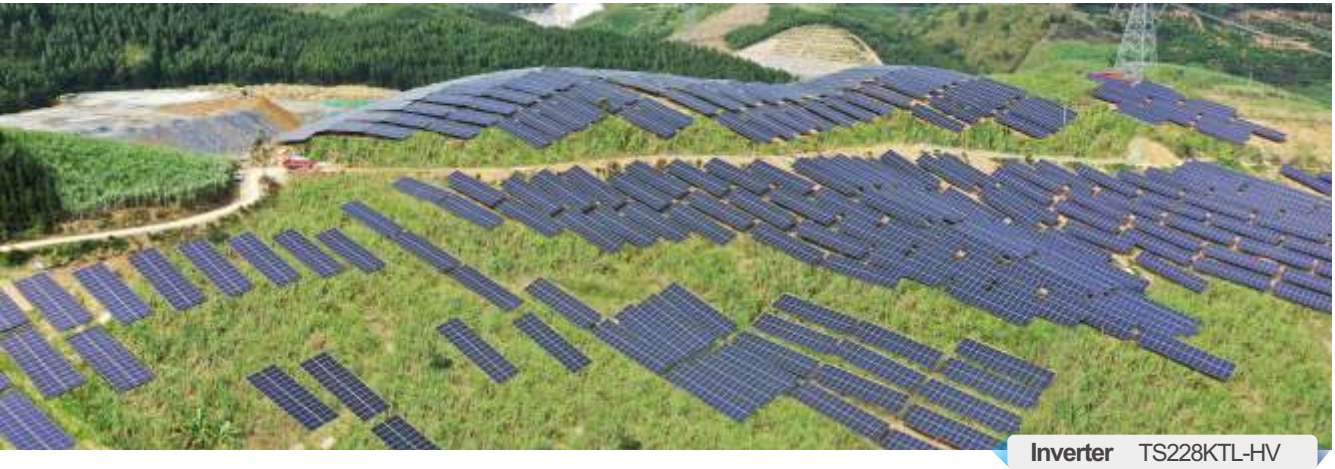
Guangxi Tianlin 60MW Photovoltaic Power Plant
